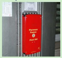
Units are available as multi or single button autodiallers providing on/dial/off functions
