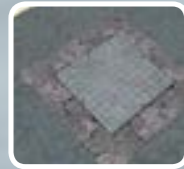
A picture frame is marked around the manhole
