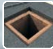
Old bedding mortar, loose bricks and debris are removed
