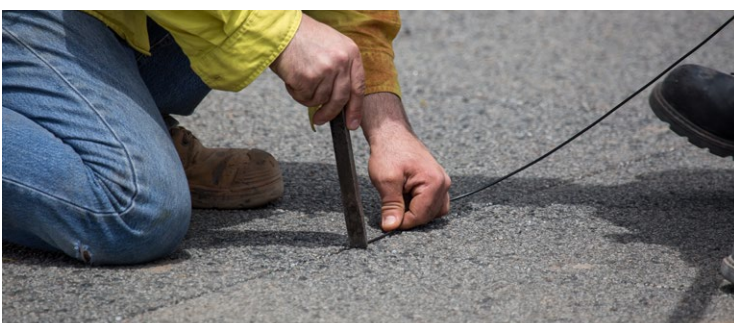
Installation of inductive loops to MetroCount specifications.
