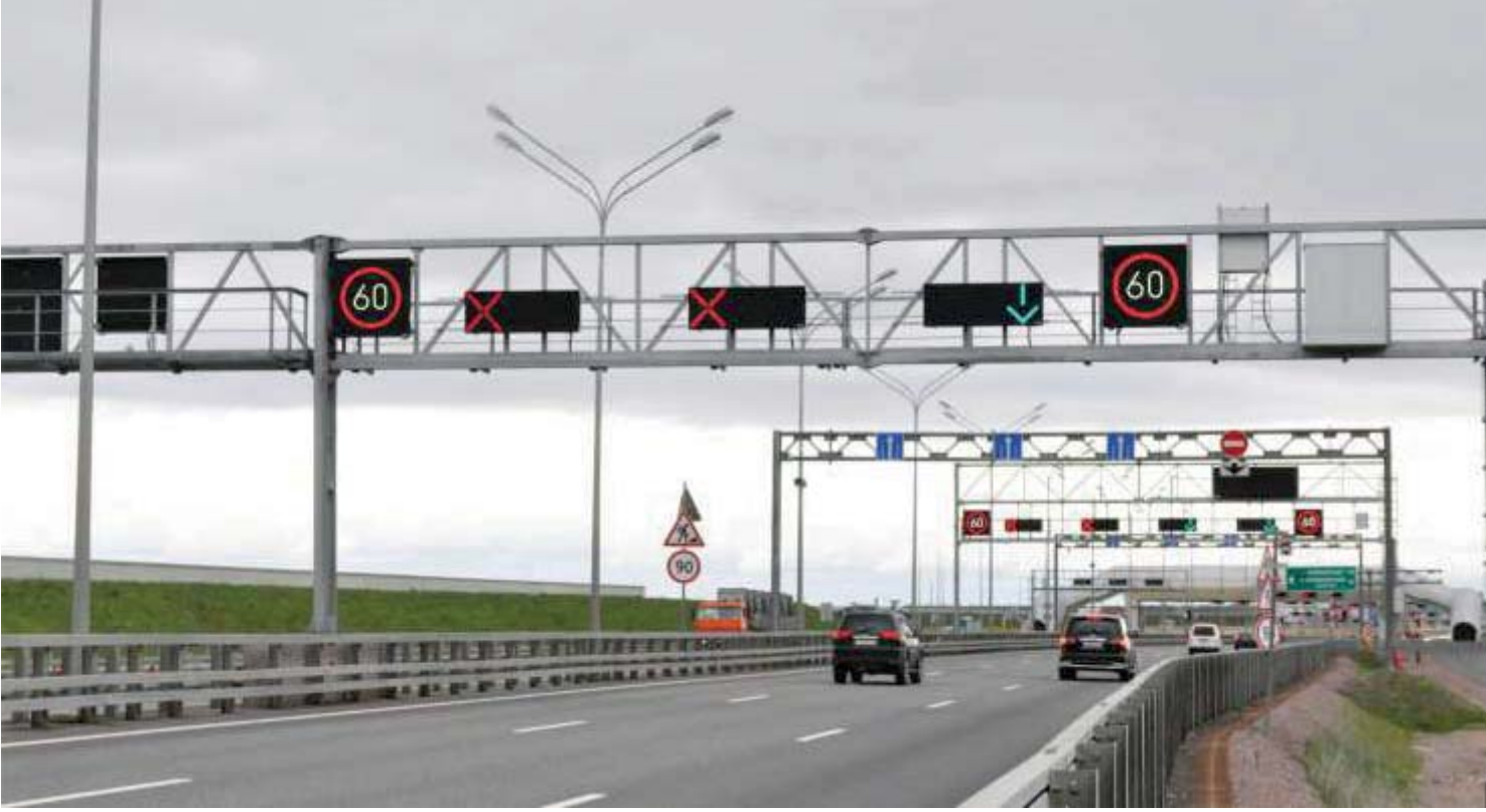
St. Petersburg Sea Tunnel, VTS, RUSSIA / 2011 St. Petersburg Deniz Tüneli, VTS, RUSYA
