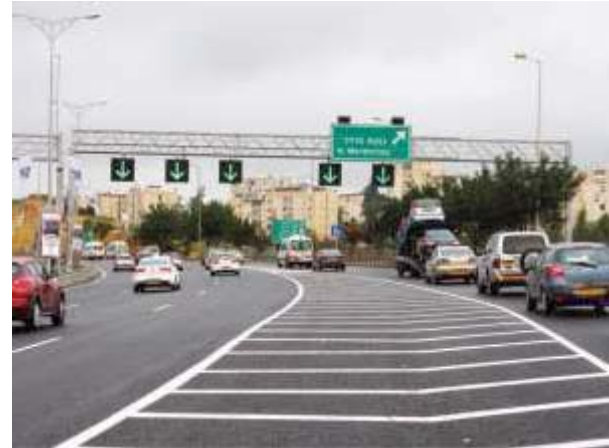
Jarusalem Begin Tunnel, VTS, ISRAEL / 2012 Kudüs Begin Tüneli, VTS, İSRAİL
