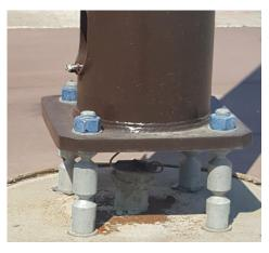
The unique physical properties and breakaway performance of Pole-Safe® gives designers greater flexibility in sizing poles.
