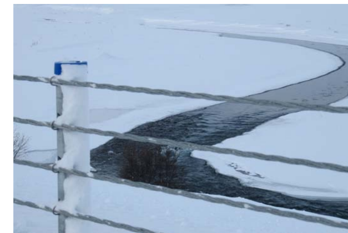
SAFENCE has proven to be very effective in snow and sand without causing drifts to settle around the road restraint system.
