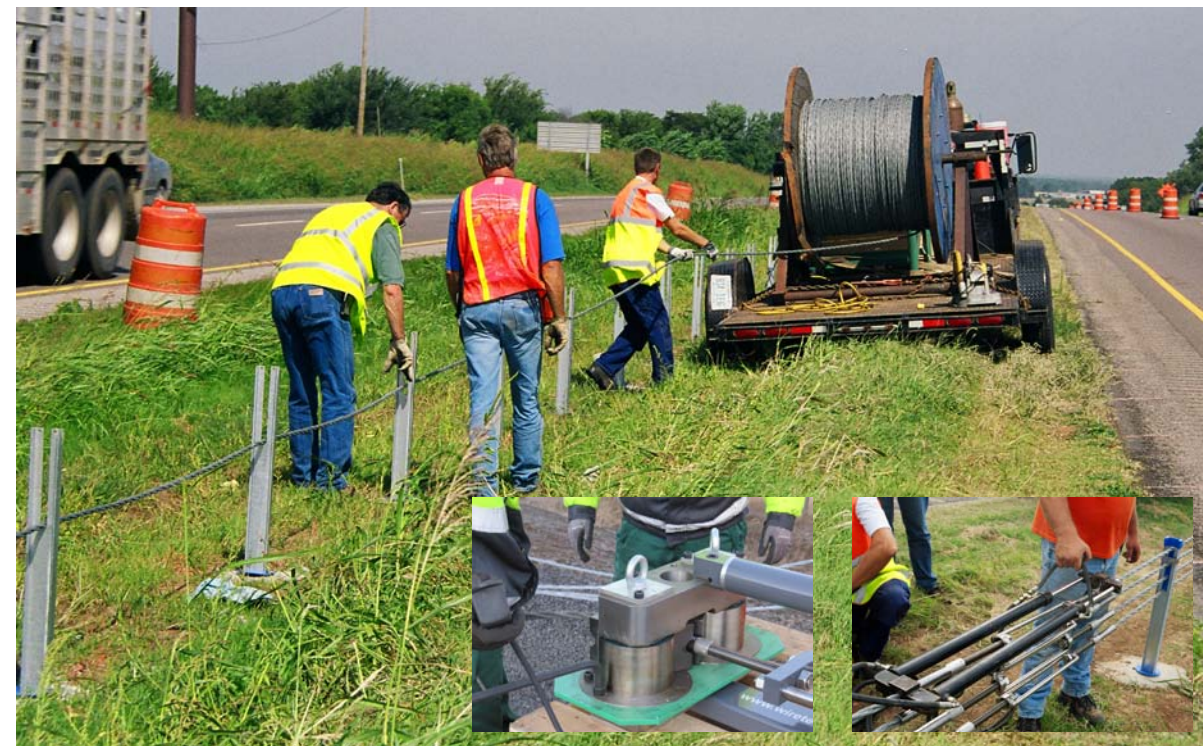
3. Wire rope is mounted and end fittings are swaged on site. SAFENCE Wire Rope Safety Fence is ready to save lives in just a few steps!
