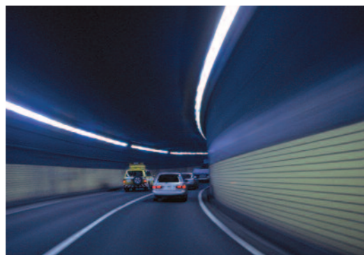
Automatic Incident Detection in tunnel
