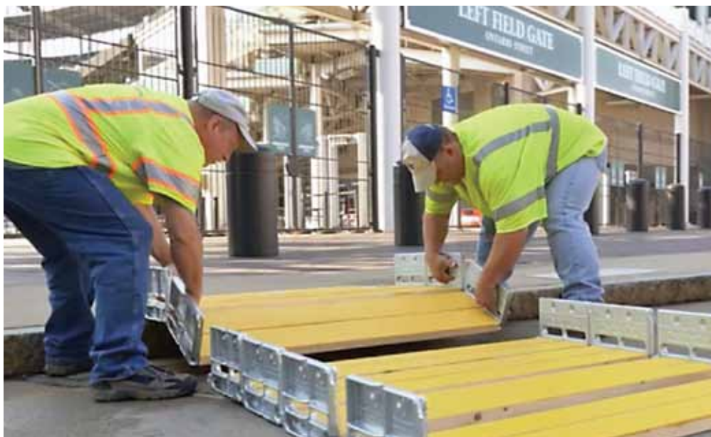
Modular sections connect for ramp length needed. No hardware required.
