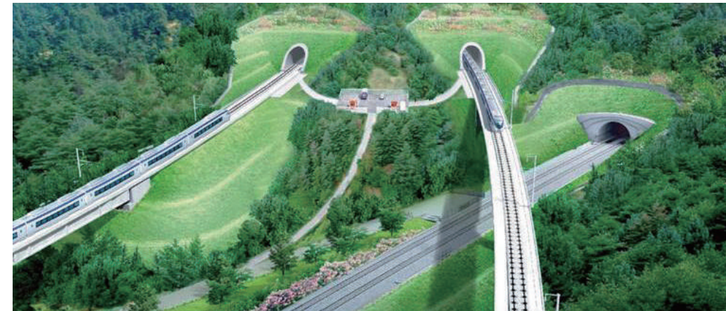
Construction Supervision services for Bujeon~Masan Double Track Railway[Lot No.4,5], Korea Length : 13.5km, Station : 1EA, Earthwork : 4.6km, Bridge : 3.0km(14ea), Tunnel : 5.9km(2ea)
