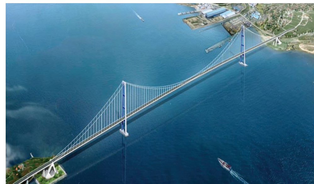
Izmit Bay Bridge on Gebze-Orhangazi-Bursa-Izmir Motorway, Turkey: - 3-span continuous bridge (L=2,800m, main span 1,550m) - Tender Design for the EPC Contractors [Nömayg JV / Hyundai E&C]
