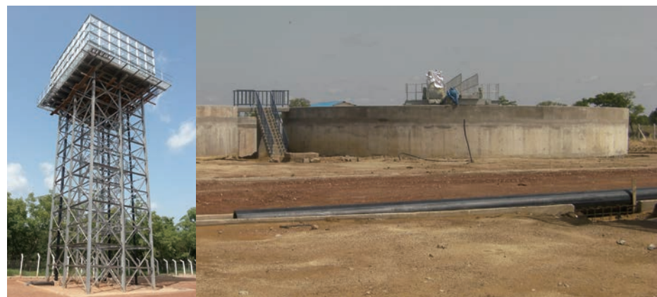
Wa City Water Supply Project, Ghana: Feasibility Study and EPC Detailed Design Intake 16,500 m 3 /day, Treatment Plant 15,000m 3 /day; Transmission Line 35km, Distribution line 99km. Public water taps: 150 places. (In Ghana, we also carried out Water Supply FS for the Cities of Techiman and Secondi-Takoradi)
