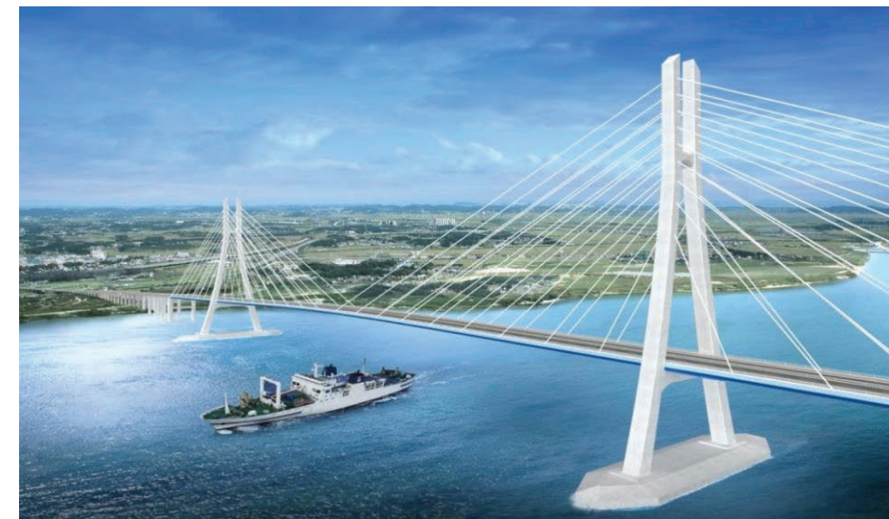
Detailed Design and Construction of Vamcong Bridge Project, Vietnam: The main bridge with 3-span continuous composite girder cable-stayed bridge (main bridge span arrangement: 210+450+210=870m). Total length of the river crossing 2.97km.
