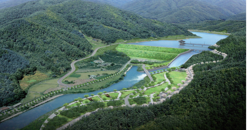
Consulting Service for Detailed Design and Construction Supervision for DauntriDam Development project, Cambodia Water supply ; 264.35 \times 106\text{m}^3/\text{yr} (Irrigation water 232.79 \times 106\text{m}^3/\text{yr} , River maintenance water 31.56 \times 106\text{m}^3/\text{yr} ) Flood control ; Maximum inflow(design flood, 1,178.4\text{m}^3/\text{sec} ), Maximum outflow : 696.9 \text{ m}^3/\text{sec} , Maximum reduction amount : 481.5 \text{ m}^3/\text{sec}
