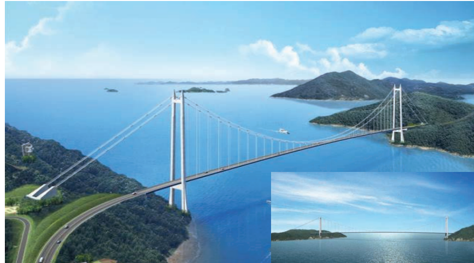
Hwayang Grand Bridge to Naro Space Center, linking Hwayang and Jukkeum Island, Korea: -Turn-key Basic Design, Main Suspension Bridge Span 810m, B=12.7m
