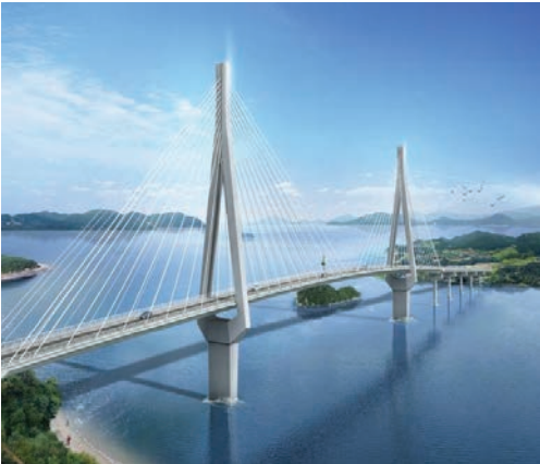
Anjwa Grand Bridge, Korea: Turn-key Basic Design, Span: 90+200+90+5@50m, Stiffening Girder: PSC Box Type
