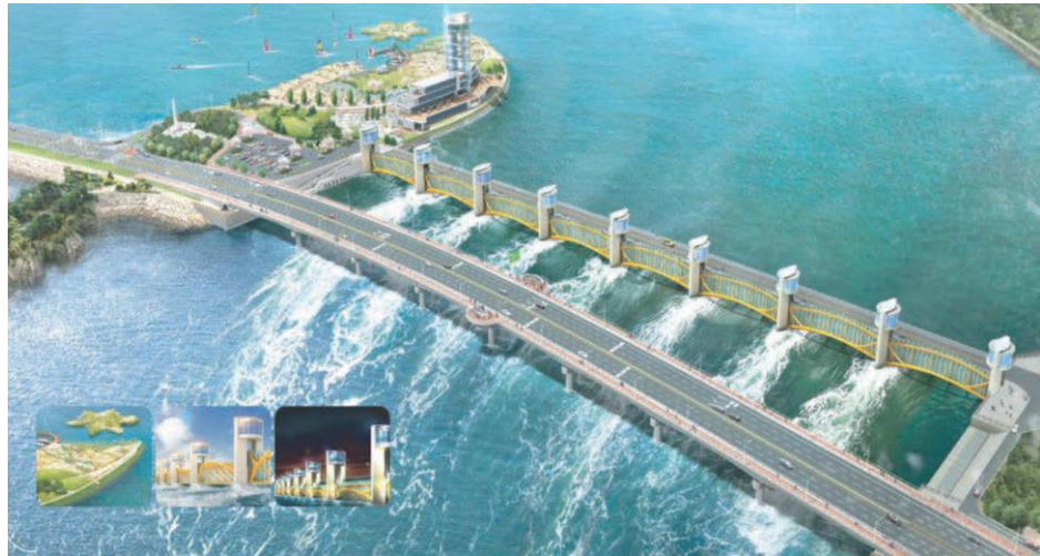
Structural Improvement of Yeongsan River Estuary Barrage, Korea - Drainage Sluice Gates 41.5m(B) x 11.1m(H) x 8 = 332.0m; - Road Bridge (36.5m x 374.3m) at seaside of drainage sluice gates; - Flood Drainage Channel: 368.0m x 1,563m (Seaside: 591m / Lakeside: 972m); - Foot Bridge: 11.0m(B)x46.0m(H)x8 = 368m (Landscape lighting and flood control telemetry system)
