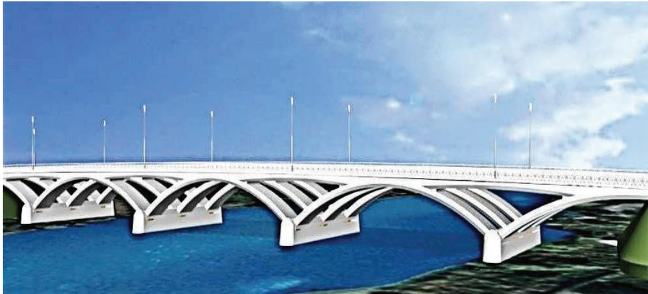
Mtskheta Bridge on Aragvi River, Georgia: Design of a 150m, 4-lane carriageway road bridge
