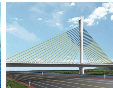
Design & Construction of Mtkvari Bridge, Tbilisi, Georgia: Asymmetric concrete cable-stayed bridge. Span = 200m, girder w = 32.0m; Interchange, ramps & landscaping
