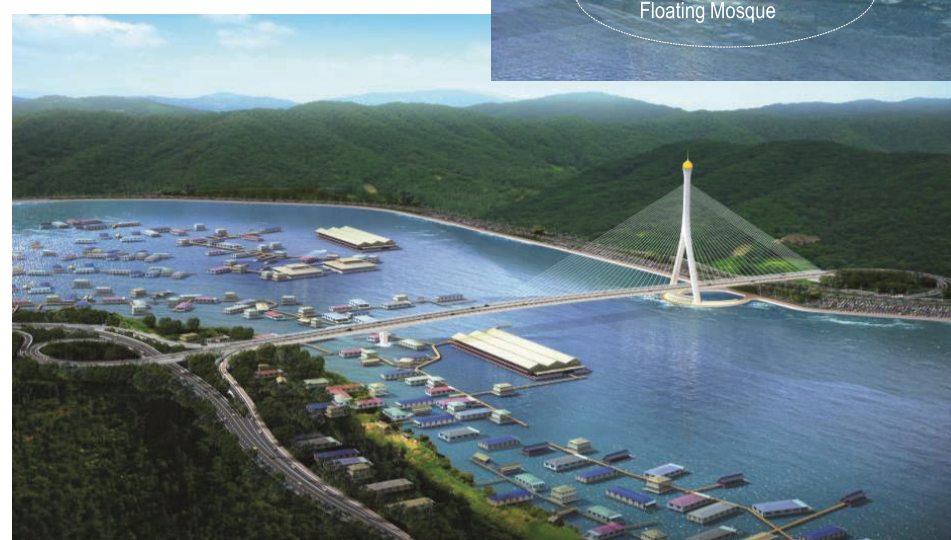
Sungai Brunei Bridge, Brunei Darussalam: New symbol of Brunei with a Floating Mosque - Client: Daelim Industrial Co., Ltd. / Employer: MOD, Brunei Darussalam - This bridge is the 2 nd longest concrete cable-stayed bridge with a single pylon in the world. - Span Arrangement: 40+87+300 (main span) + 180 = 607m - Stiffening Girder: One-cell Concrete Box Girder / Concrete Pylons / FCM Construction - The bridge features a unique Floating Mosque at its Substructure
