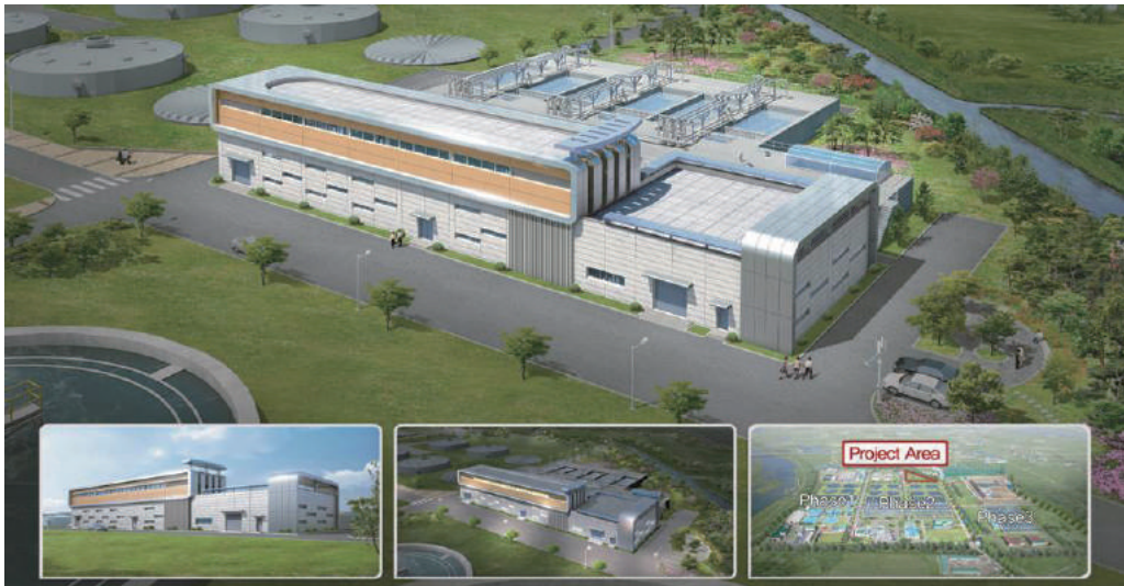
Jeonju Advanced Sewage Treatment (T-P Removal) Plant, Korea: Basic & Detailed Design on the turn-key basis (403,000m³/day, ACTIFLO Process)
