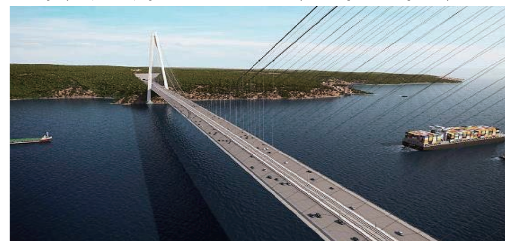
The Third Bosphorus Bridge, Istanbul, Turkey: Tender Design and Implementation Design for the Contractors - Location: Bosphorus Garipce - Poyraz, Istandub; 3-span continuous bridge (L=1,598m, Main Span = 1,645m - Illustration above is the artist's impression of the project at the time of the tender design
