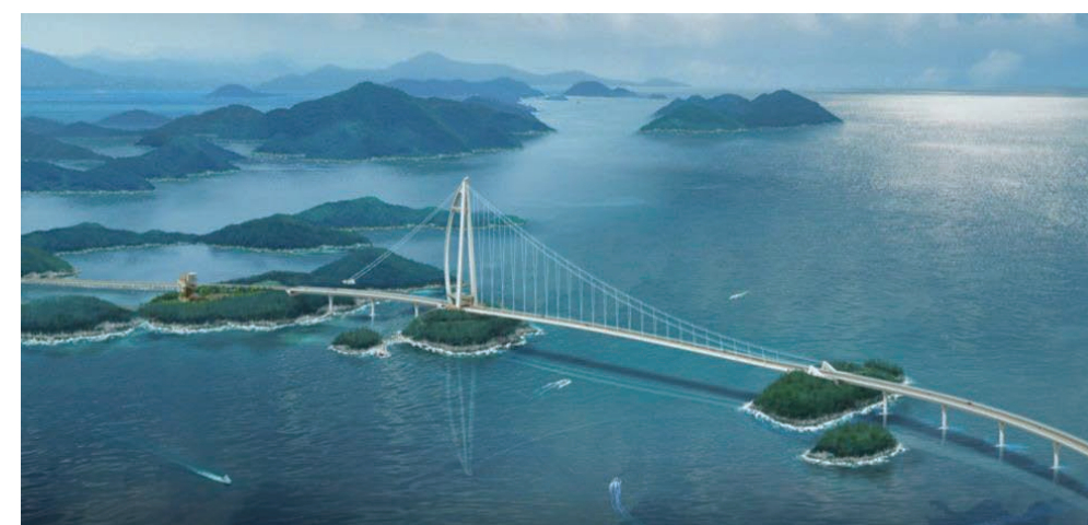
Dandeung Bridge on Gogunsan Islands Link Road, Korea: - Turn-key Basic & Detailed Design - Single Pylon with 400 m Main Span, B=20m - D-shape Pylon (H=105m) represents a sail hoisted to a boat, symbolizing local fishing industry
