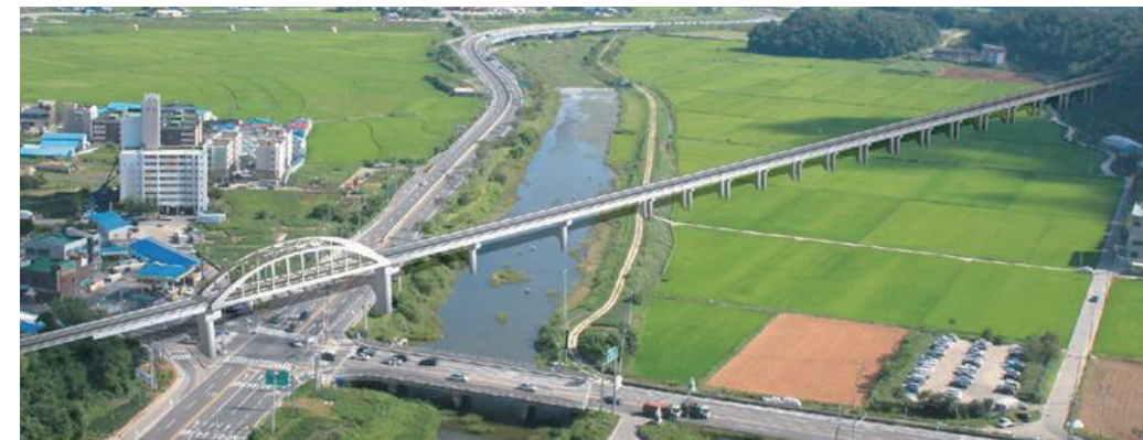
Detailed Design for improvement in Janghang line [Phase 2, Lot No. 1], Korea Length : 18.3km, Station : 1EA, Earthwork : 12.7km, Bridge : 4.5km(13ea), Tunnel : 1.1km(2ea)
