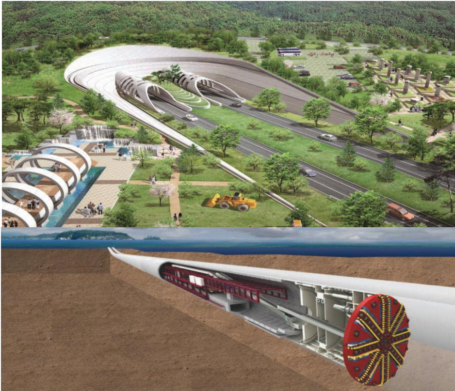
Construction of Boryung - Taejeon Highway - Lot 1, Korea: 1) Design of TBM tunnel portal area landscaping plan; and 2) Design of Shield TBM Tunnel (Length = 6.9km) at Under-sea Tunnel Section on the Highway Lot 1 Section
