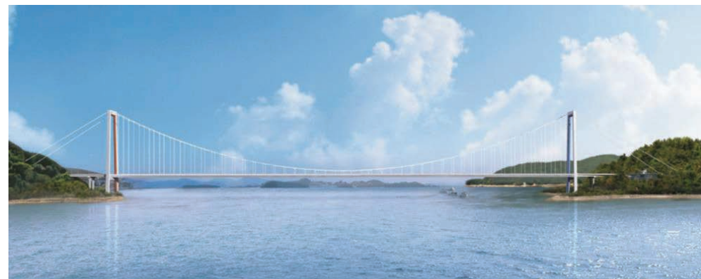
The Second Namhae Bridge, Korea: -Alternative tender design single span suspension bridge (Main span=815m, B=24.5m)
