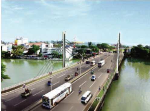
Mahanama Bridge, Sri Lanka: Turnkey Design of Cable-stayed bridge with PSC Beam girder
