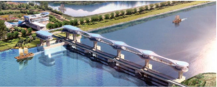
The Yeongsan River Improvement Project - Section 2 (Dasi District), Korea: River improvement of 12.29km; with movable weir 184m; water gates (L=36.5m, H=7.13m); Spillway bridge (L=622m, B=5.34m); Stop-log bridge (L=235m, B=5.3m); Small hydro plant (610kw x 2ea); Bicycle lane, ecology park, cultural and leisure spaces, etc.
