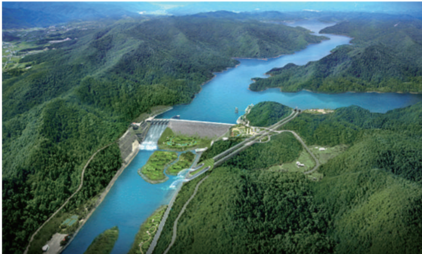
Detailed Design (Turn-Key) for Juam-dam waterway: tunnel Construction Project, Korea Water conduction tunnel : 11.23km ; TBM(Tunnel Boring Machine Method, 10.913km) NATM(New Austrian Tunneling Method, 0.317km) Intake tower 2ea ; (B 3.3m × H 3.3m × 2ea, entrance & outlet section), etc
