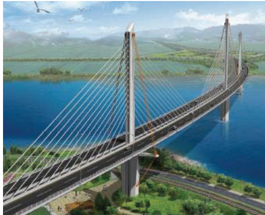
Sepoong Bridge on Sepoong-Junggun Bypass, Korea: Alternative Design and Detailed Design. Span: 57.5+85+2@220+85+57.5=725 m
