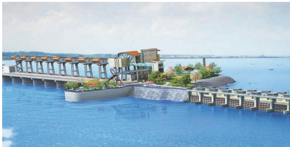
Drainage Sluice Gate Expansion of Asan Bay Tidal Barrage, Korea The project is to prevent sea water intrusion, and preserve irrigation water for farmland by improvement and upgrading of structures including sluice gates and bridge
