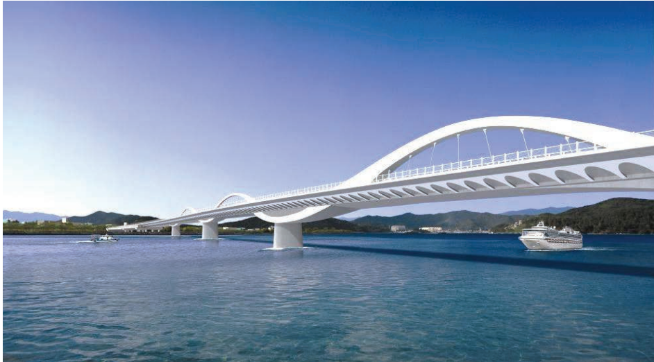
Angol Multi-span Arch Bridge as a New Landmark of Busan New Port at Angol Bay, Korea: Multip-span arches of 110m each with Parallel strand system & FCM construction.
