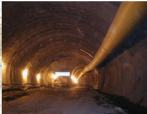
Youngdong Railway Line Dongbaeksan – Dogye Alignment Relocation Project, Korea: New alignment construction of 17.78km including 15.9km NATM tunnel and two new stations.
