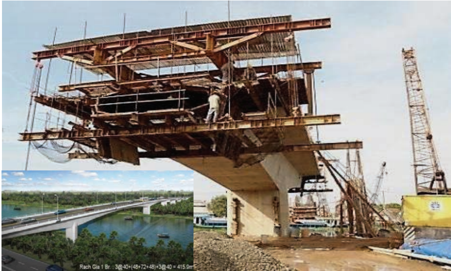
GMS-SCCP Rach Gia Bypass Project, Vietnam: Bypass 20.83km with 22 bridges (3,234m total); Bridge Types: PC Voided Slab, PC I-girder, Super T-girder, PC Box girder; Foundation: CIP Concrete Piles of bored & cast in situ, Precast RC Piles); Extensive soft-soil treatment.
