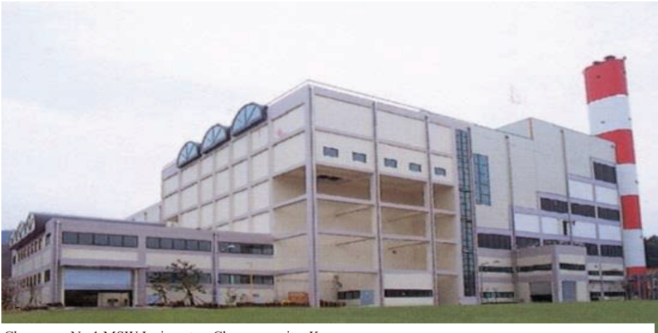
Changwon No.1 MSW Incinerator, Changwon city, Korea - Incinerator type: Stoker; Capacity: 200 ton/day; Turbine Generator : 1,100kW
