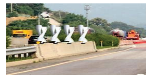
Roadside Wind Turbines convert turbulence from high-speed traffic to electricity for smart highway equipment
