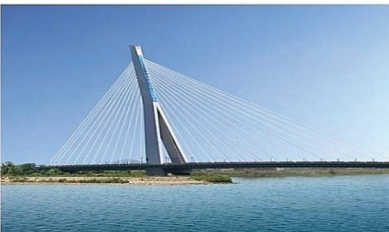
Construction of Gongchon I Bridge, Incheon, Korea: Design and Implementation Methods Services for Asymmetric 15-degree Inclined Pylon (109m) Cable Stayed Bridge (300m long with 6-lane)
