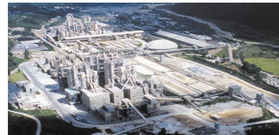
Kiln Waste Heat Recovery Power Plant for Ssangyong Cement Factory, Korea: Basic and Detailed Design. Steam Production 190.8 ton/hr; Power Generation 43.5 MW; Steam Turbine (1 unit); AQC Boiler (4 units); PH Boiler (7 units)
