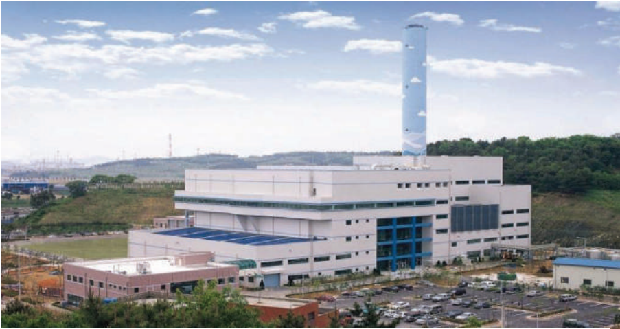
Ulsan Municipal Solid Waste Incinerator, Ulsan city, Korea - Incinerator type: Stoker / Capacity: 200 ton/day x 2 / Turbine Generator : 1,500kW
