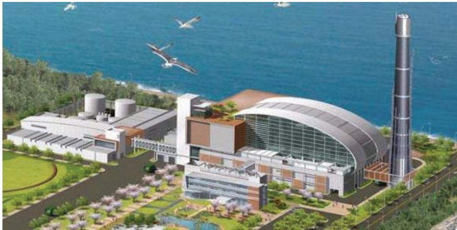
Songdo Food Waste Treatment Plant, Korea: - Capacity: Food Waste 200 ton/day, Feedstuff 32ton/day
