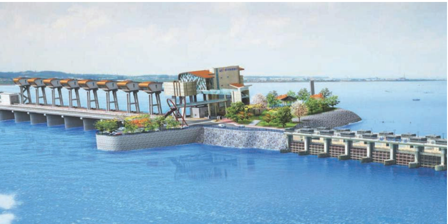
Drainage Sluice Gate Expansion of Asan Bay Tidal Barrage, Korea: Agricultural irrigation/drainage infrastructure for prevention of sea water intrusion comprising construction of drainage sluice gates, expansion and upgrading of bridge.
