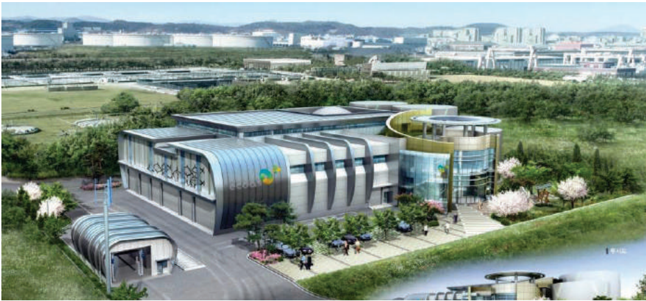
Organic Waste to Bio-gas Facility, Ulsan City, Korea: - Treatment Process : Anaerobic Digestion & Composting - Capacity: 150 ton/day (Food Waste 100 ton/day / Livestock Manure 50 ton/day) - Bio-gas: 9,446 Nm³/day; Steam: 4 ton/h
