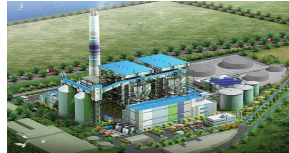
Technical Audit on Improvement of Yeosu Co-generation Plant, Korea Southeast Power Co.: Condensing Turbine: 67.9MW (1 unit); Back Pressure Turbine: 24.4MW (2 units); Boiler: CFBC 350ton/hour (2 units)
