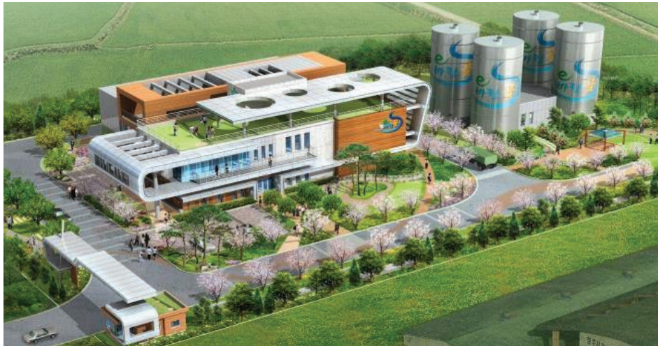
Cheongju Food Wastewater to Bio-gas Facility, Korea: - Treatment Process : Anaerobic Digestion & Electricity Generation - Capacity : Food wastewater 200 ton/day for power generation of 708 kW
