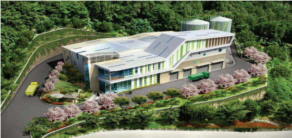
Organic Waste to Bio-gas Facility, Yangsan City, Korea: - Treatment Process : Anaerobic Digestion & Electricity Generation - Capacity : Food Waste 60 ton/day / Livestock Manure 70 ton/day - Biogas 6,196Nm³/day and Generation: 534 kW
