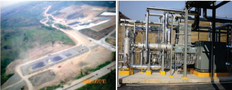
Bulacan LFG Collection & Power Generation Project, the Philippines: Feasibility Study Site Area: 40ha; Capacity: 2000 ton/day for 20 years; Expected Growth Power Generation: 5MW
