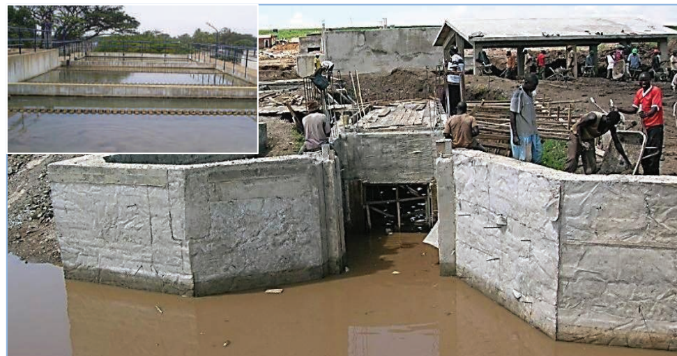
Awendo Region Drinking Water Development Project, Kenya: PMC service from preparation and implementation of the project to improve hygienic conditions of African rural communities. Project components comprised intake weir and conveyance line 3km, treatment (2,000m 3 /day) and storage (1,000m 3 ), treated water conveyance (7km), distribution (15km), and deep-well drillings (2) with 5 distribution kiosks.
