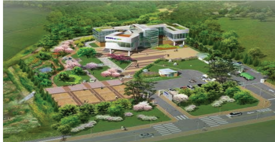
Chungbuk Water Quality Restoration Center, Pyungtaek City, Korea: Treatment Type: DFS-MBR; Capacity: 8,200 + 800 m 3 /day / Recycling Water 2,800m 3 /day
