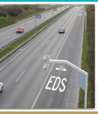
Hard shoulder enforcement system, by sensing the vehicles moving on the safety lane, performs violation detection. Entirely automatic system takes the photo of violating vehicles and transmits them to the center.
