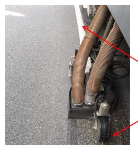
Smets ARC system in operation on a road (removing road lines).
