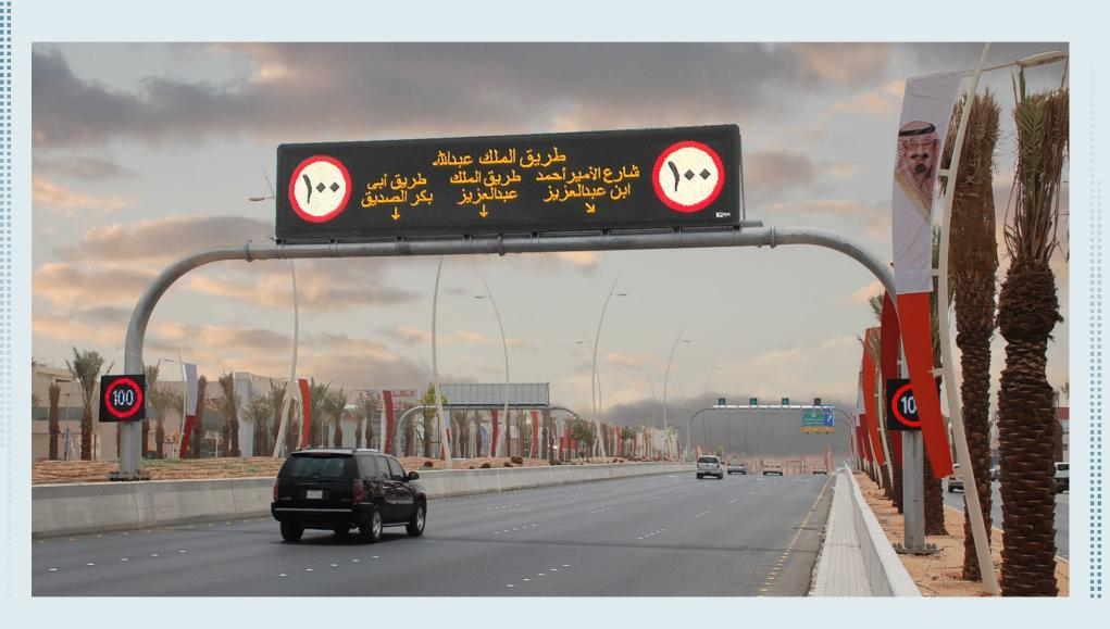
Variable message signs can be placed in a wide range of places like highways, urban arteries, and major road junctions. Typically installed at the side or above the roadway, the VMS uses text and graphics in monochrome or color format to inform drivers of a variety of situations including emergencies, construction, and delays. Our variable message signs come in two major formats:
