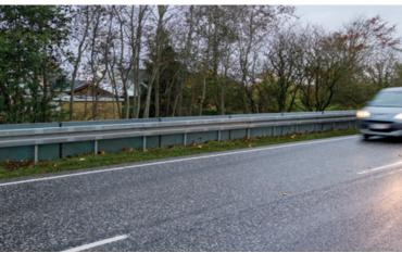
cles. With a sound source that low, there is no need for a massive wall to block the noise, if a screen can be brought close enough to the traffic. The solution is the noise absorbing safety barrier EasyRail® NA.
