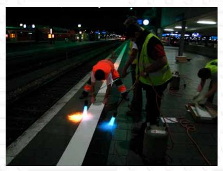
enables the products to follow the existing contours of all surfaces. The installation only requires a broom, a propane burner and a roller.
